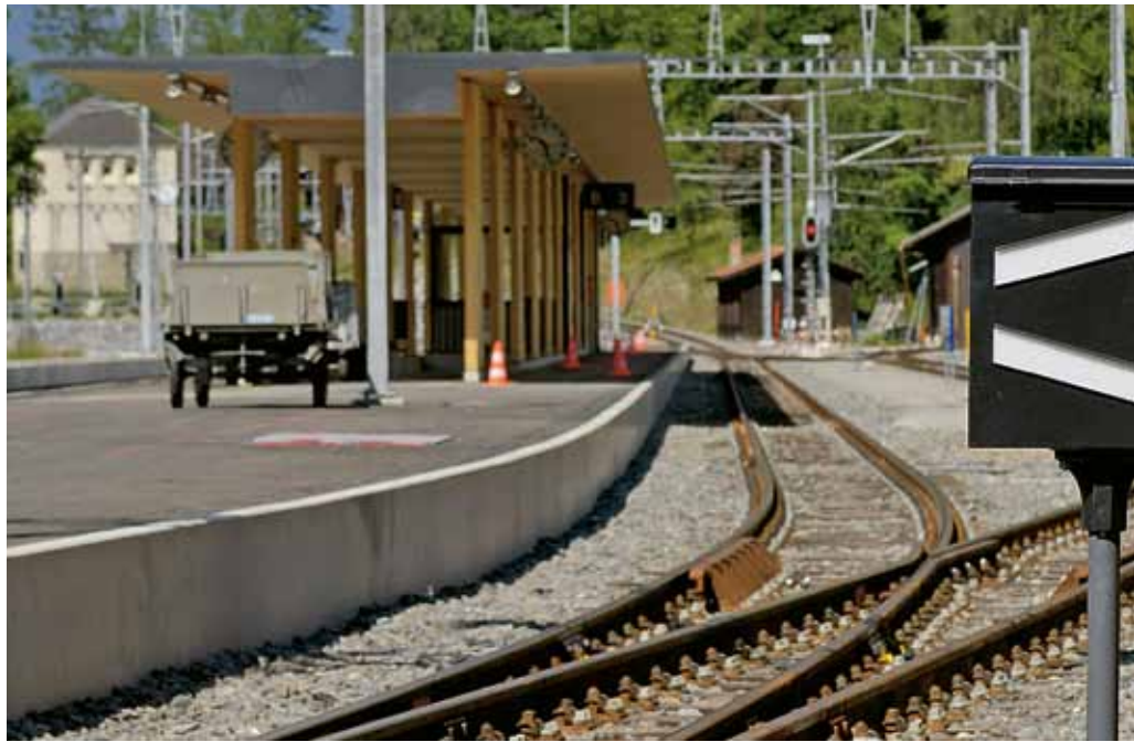
State-of-the-art Simis IS technology in daily application in Filisur, Rhetian Railway
